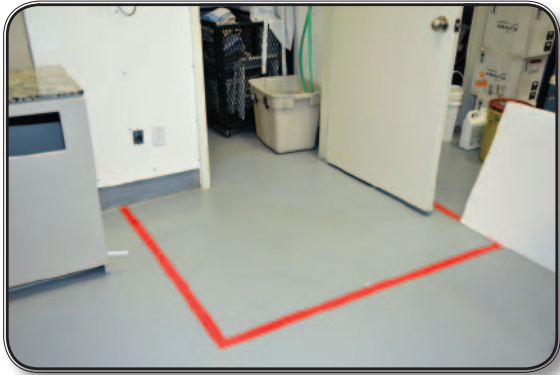
1 A demarcation line serves as a visible indicator of transitioning zones in a veterinary setting.
