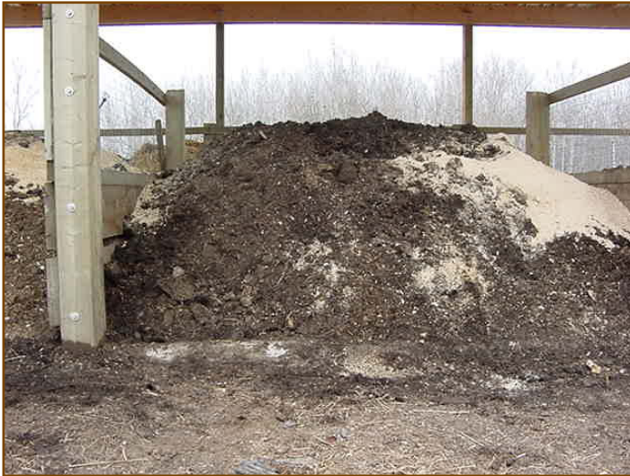
Figure 8: This bin has a concrete base with a 4 in. curb. Courtesy: Birch Bay Pork.
