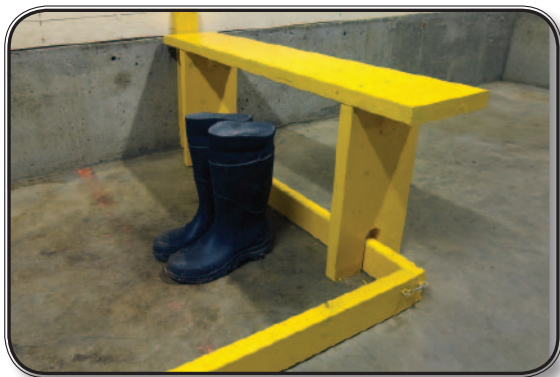
2 A crossover barrier built to size that accommodates changing footwear or donning booties by incorporating a bench into the design.
